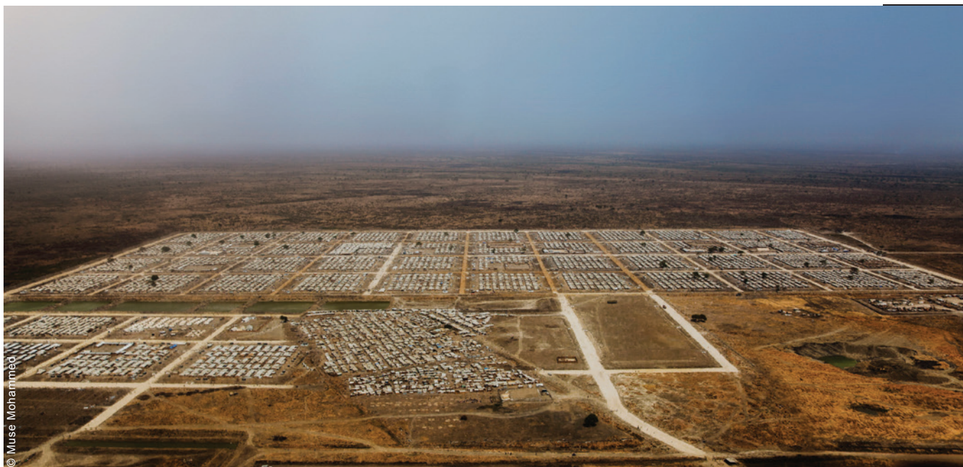
The expansion plan included land that was already spontaneously occupied by camp residents. Careful phasing of major upgrading works was required, as the whole site needed to be upgraded.
