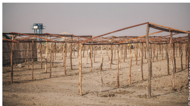
Shelter frames were built by contractors.
