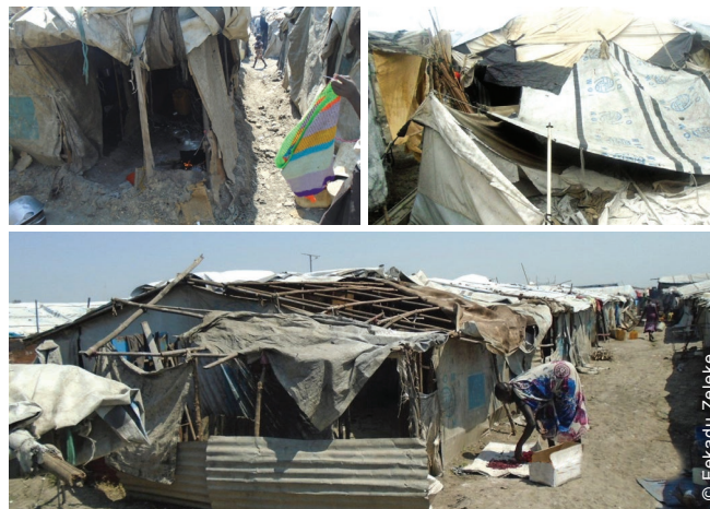
Before rehabilitation, the site offered very poor shelter conditions and was overcrowded, with related fire and safety risks for its residents.
