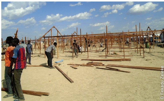
New shelters were built by local community members after ground levelling.
